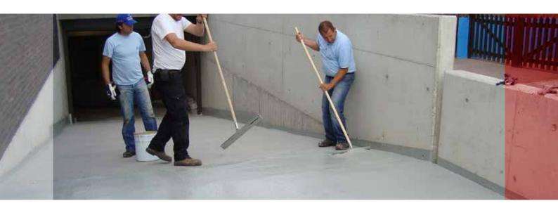
Within this range, contractors will find all kinds of products for the protection of foundations and for the curing of fresh concrete structures in road construction.
