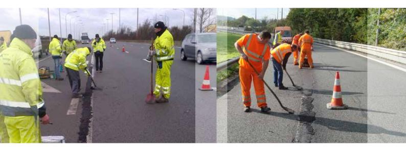
IKO road offers a very complete range of products for the repair and renovation of road surfaces. The product range includes cold asphalt in various qualities, depending on the application and the desired result.
