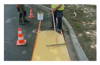
These are mainly coloured coatings, which may or may not be reflective, with very quick curing and a non-slip surface. The range also includes fast-curing adhesives to stick reflectors into the road.
