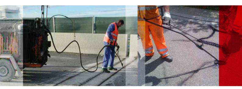
IKO road offers a whole host of products to fill (expansion) joints and cracks in road surfaces. There are products for both concrete and asphalt. These products can be used in new buildings and renovation projects.
